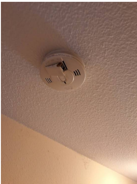
Smoke / Monoxide detector in hallway
