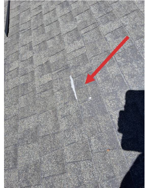
South face of roof
