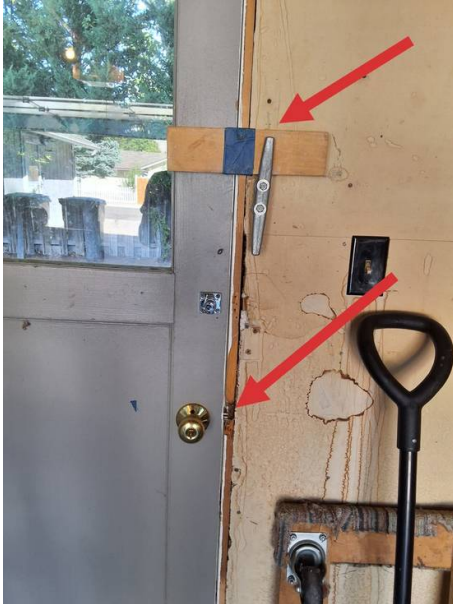
Man door at rear of garage
