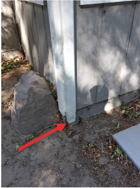
Downspout at rear of home
