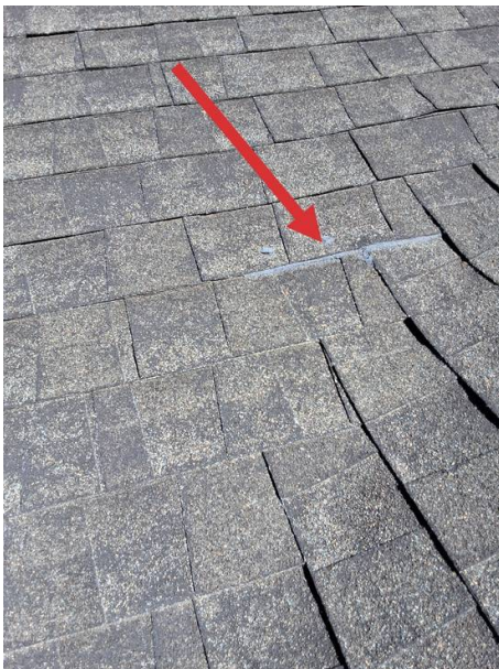
South face of roof
