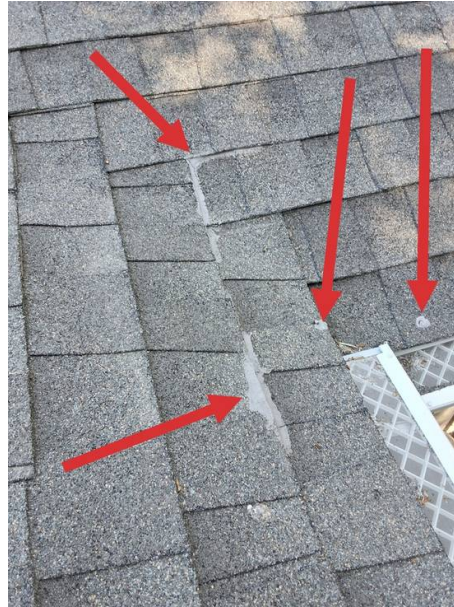
East face of roof
