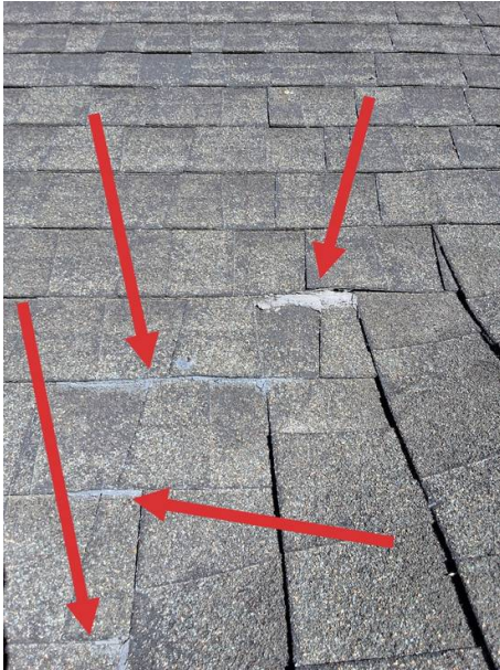
South face of roof
