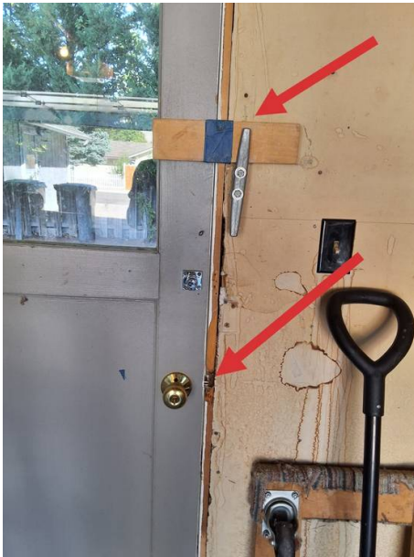
Man door at rear of garage
