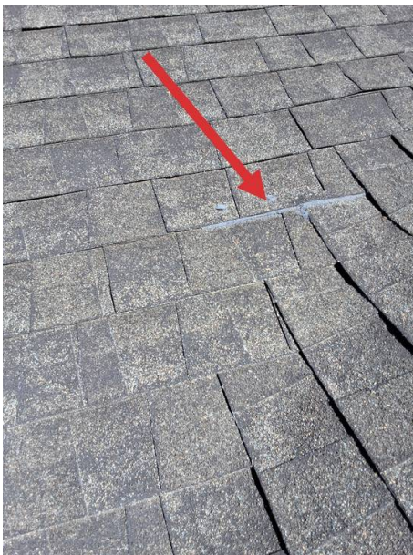
South face of roof
