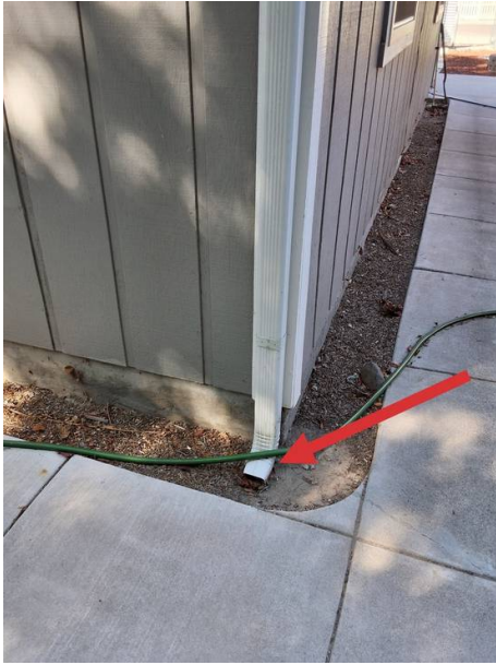
Downspout at rear of home
