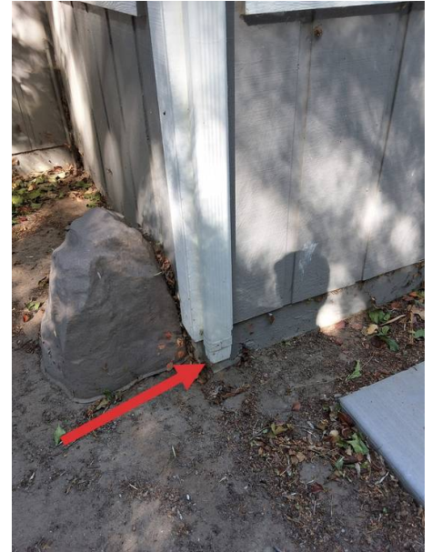
Downspout at rear of home
