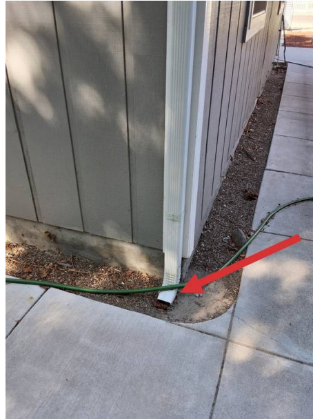
Downspout at rear of home
