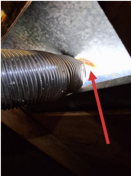
Bathroom vents terminating in attic
