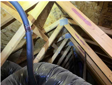
Roof Structure/Framing: Roof Structure Type Manufactured Trusses, OSB Sheathing
