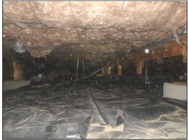
3.0 Item 4(Picture) view of crawlspace
