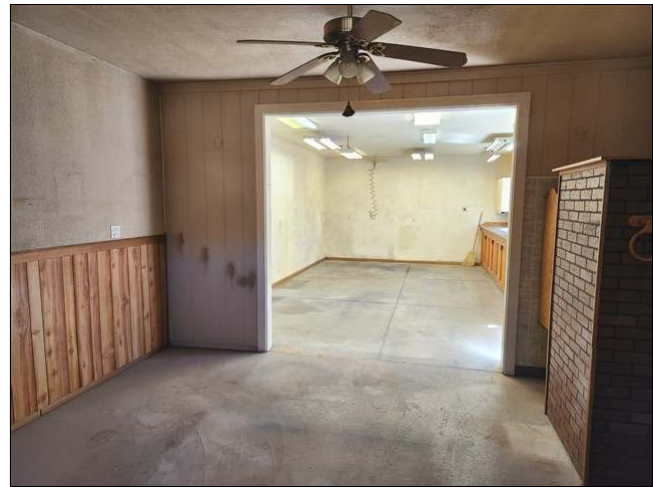
11.0 Item 2(Picture) view of workshop interior
