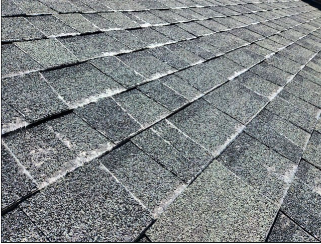
2.1 Item 1(Picture) condition of south shingles
