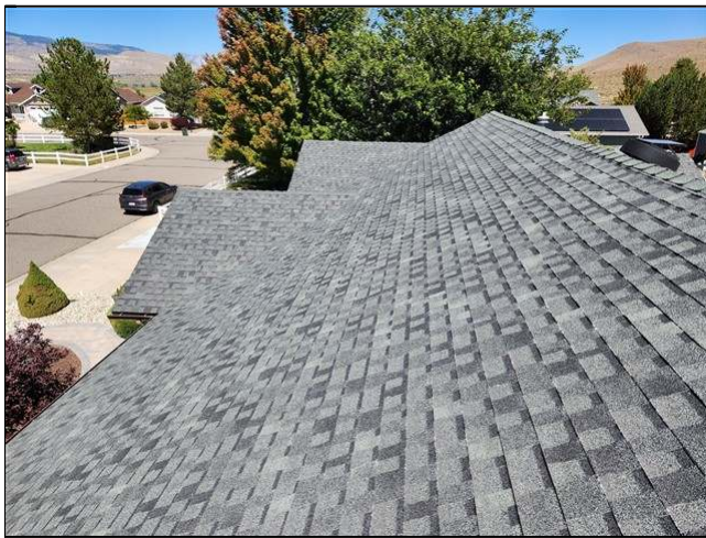
2.0 Item 1(Picture) view of roof
