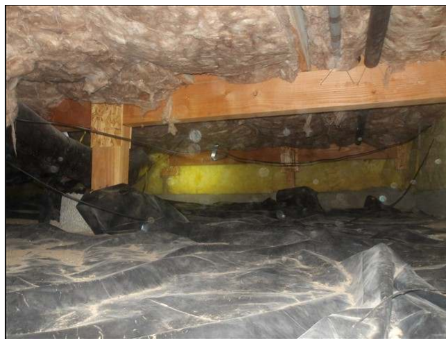
3.0 Item 2(Picture) view of crawlspace
