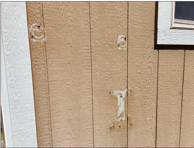
1.1 Item 1(Picture) caulking maintenance at the South wall cladding
