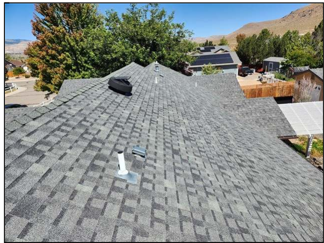
2.0 Item 2(Picture) view of roof
