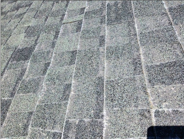
2.1 Item 3(Picture) condition of south shingles
