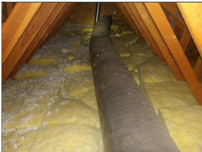
9.0 Item 3(Picture) Cathedral Ceiling Attic insulation
