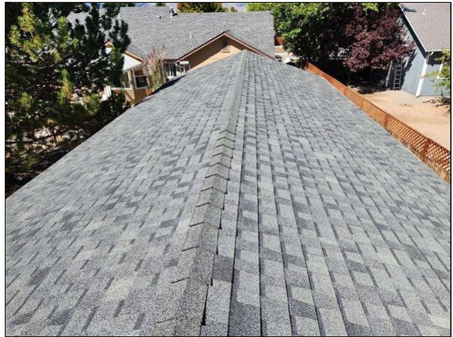
11.3 Item 2(Picture) view of roof
