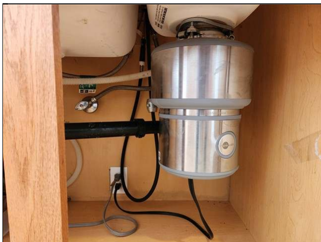
6.4 Item 1(Picture) disposer has a "delayed" start
