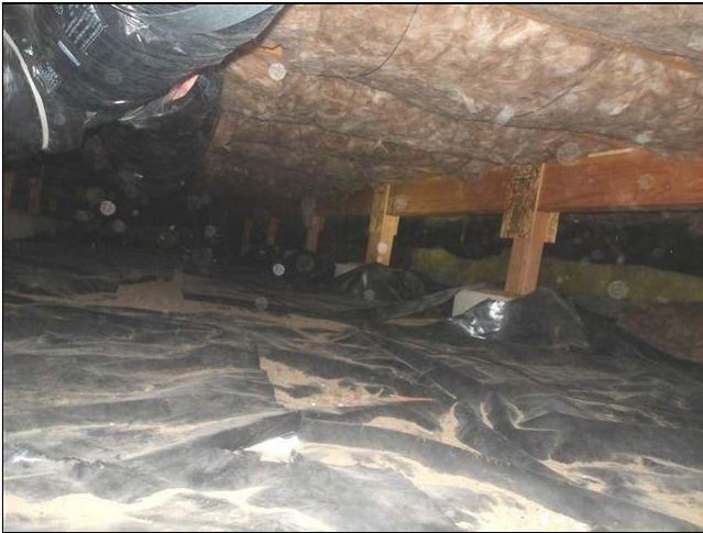
3.0 Item 5(Picture) view of crawlspace
