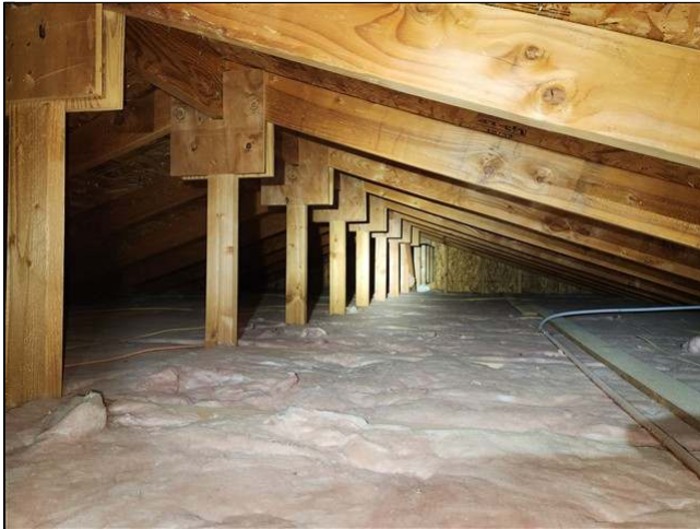
11.4 Item 1(Picture) view of rear section attic
