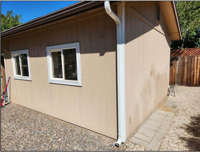
11.1 Item 1(Picture) view of exterior wall siding
