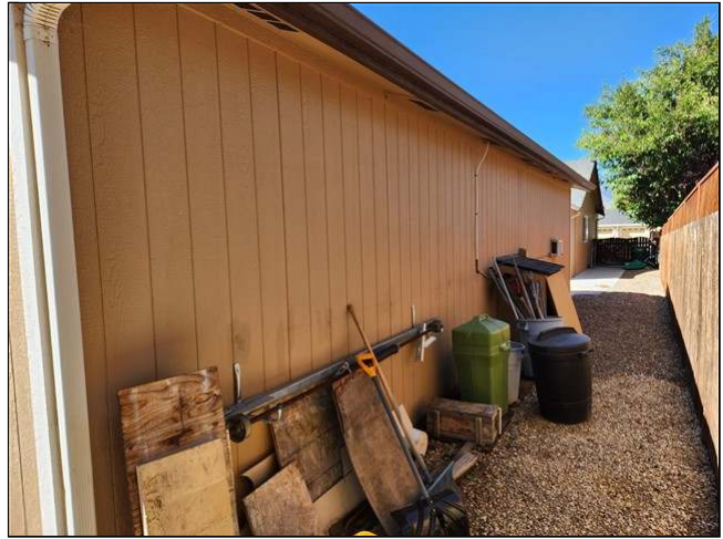
11.1 Item 2(Picture) view of exterior wall siding
