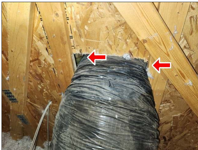
8.2 Item 1(Picture) open to the home's attic space
