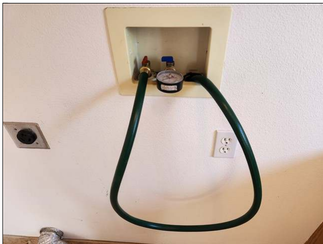
5.6 Item 1(Picture) checking laundry valves and drain
