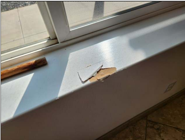
7.5 Item 1(Picture) East wall window sill board
