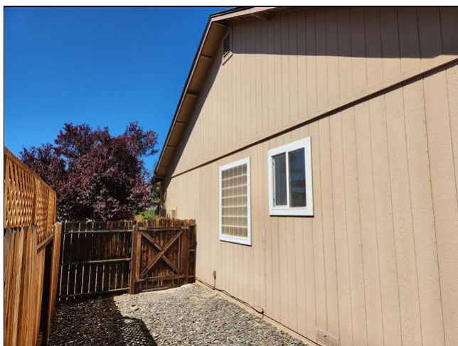
1.0 Item 1(Picture) view of exterior
