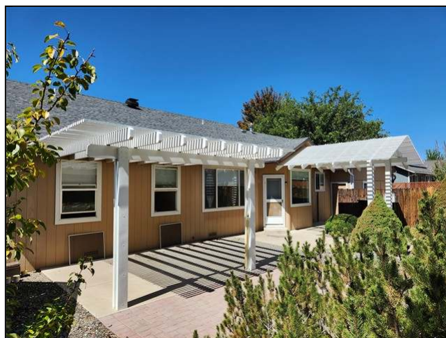
1.0 Item 2(Picture) view of exterior
