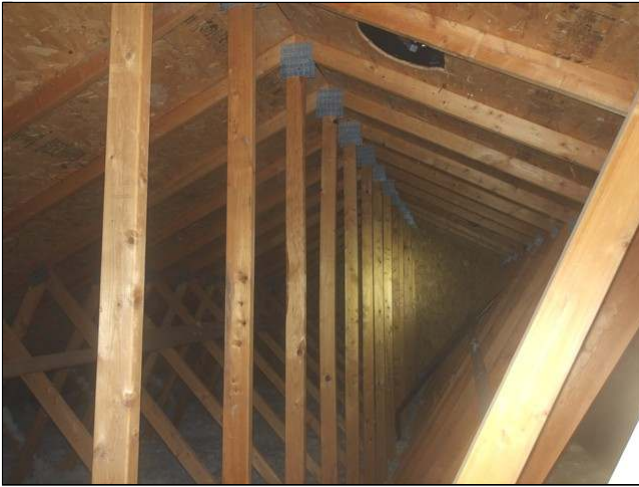
3.8 Item 1(Picture) view of attic
