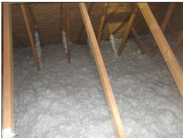
9.0 Item 1(Picture) view of attic insulation
