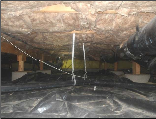
3.0 Item 3(Picture) view of crawlspace
