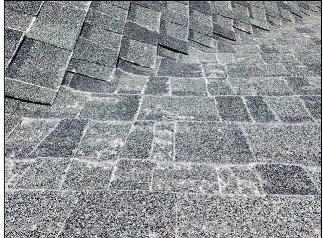
2.1 Item 4(Picture) condition of south shingles
