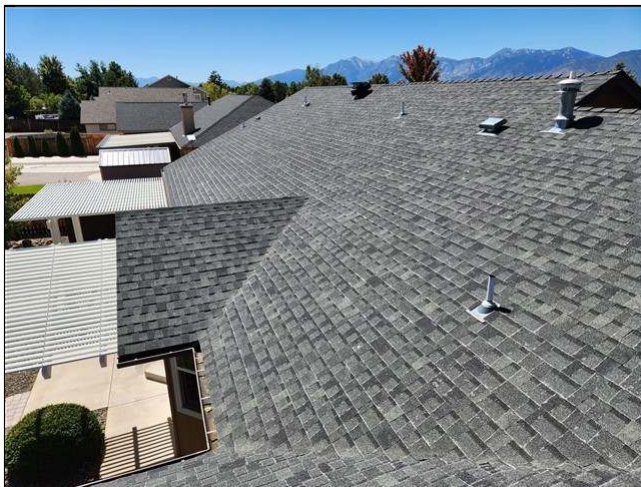
2.0 Item 3(Picture) view of roof
