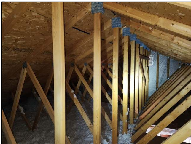
8.11 Item 3(Picture) view of garage roof structure
