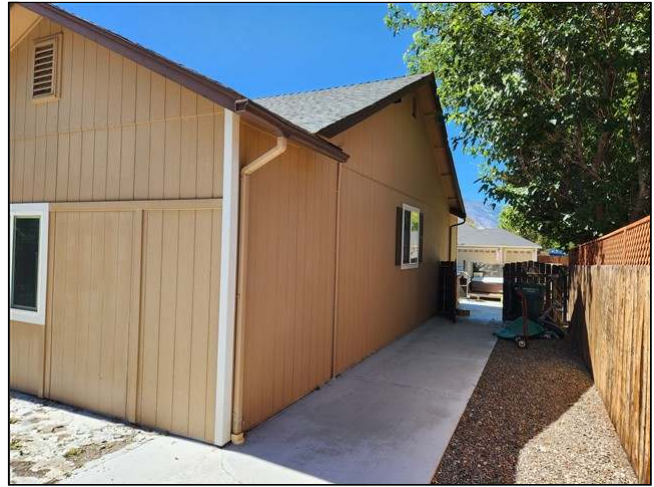
1.0 Item 4(Picture) view of exterior
