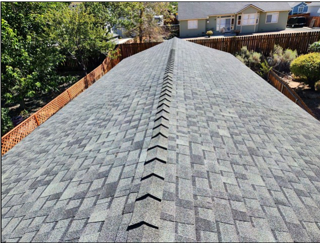
11.3 Item 1(Picture) view of roof
