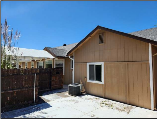
1.0 Item 3(Picture) view of exterior
