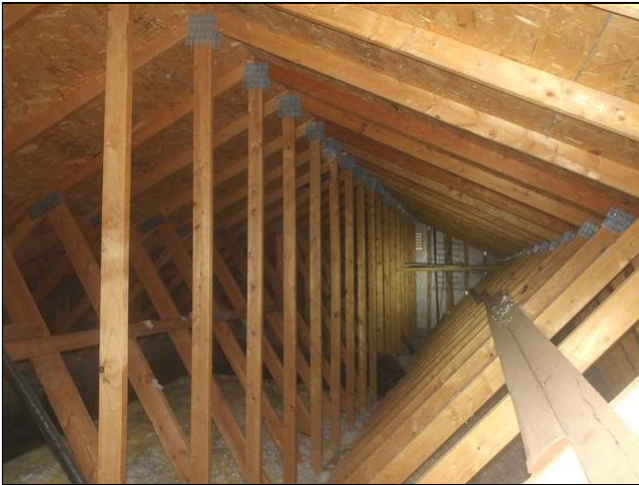
3.8 Item 3(Picture) view of attic
