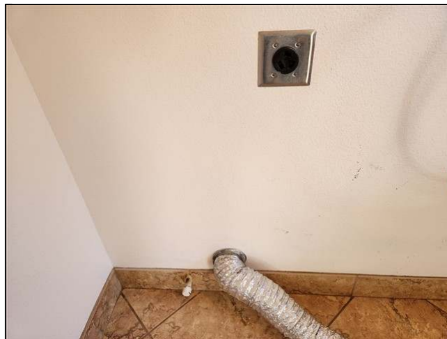
5.6 Item 2(Picture) laundry hookups
