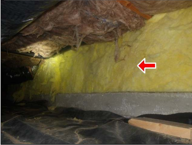
9.1 Item 1(Picture) insulated on the perimeter of the foundation
