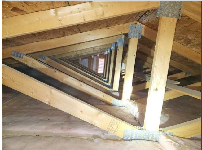
11.4 Item 2(Picture) view of front section attic
