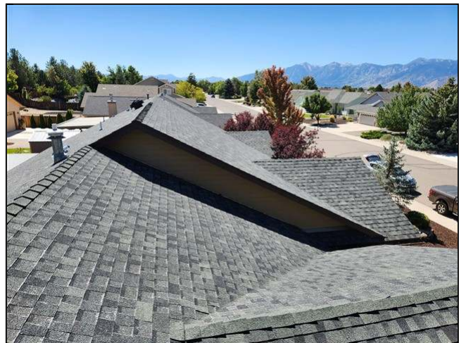
2.0 Item 4(Picture) view of roof
