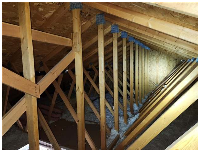
8.11 Item 2(Picture) view of garage roof structure
