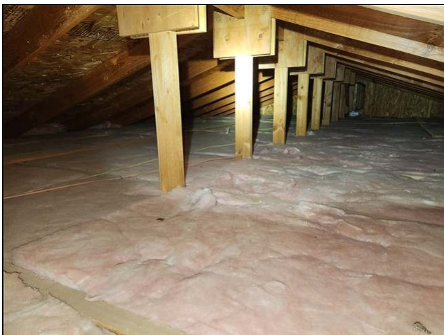
11.7 Item 1(Picture) view of attic insulation
