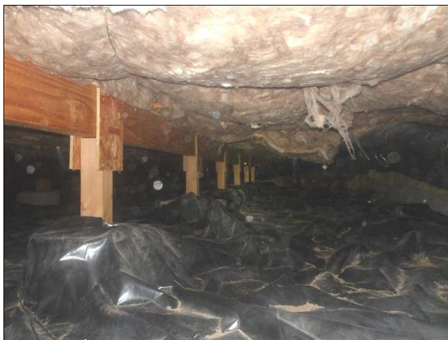
3.0 Item 1(Picture) view of crawlspace
