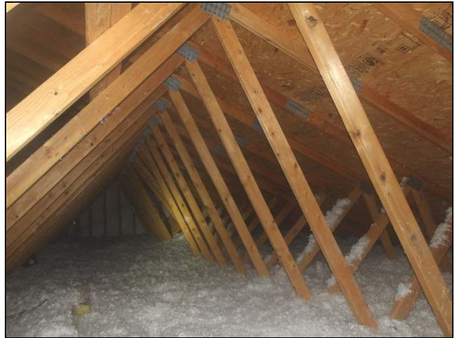
3.8 Item 4(Picture) view of attic
