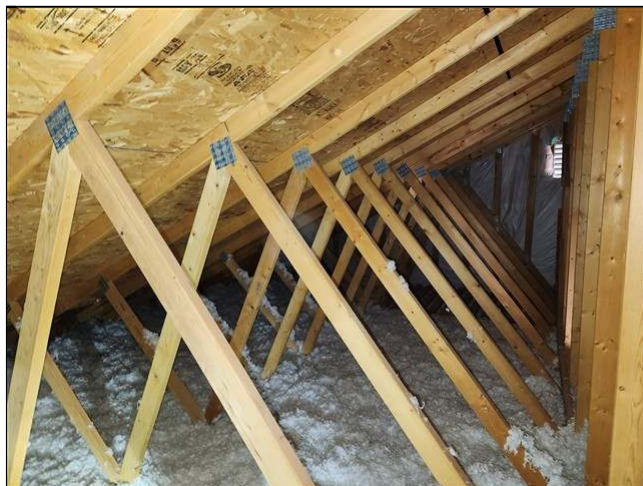
8.11 Item 4(Picture) view of garage roof structure
