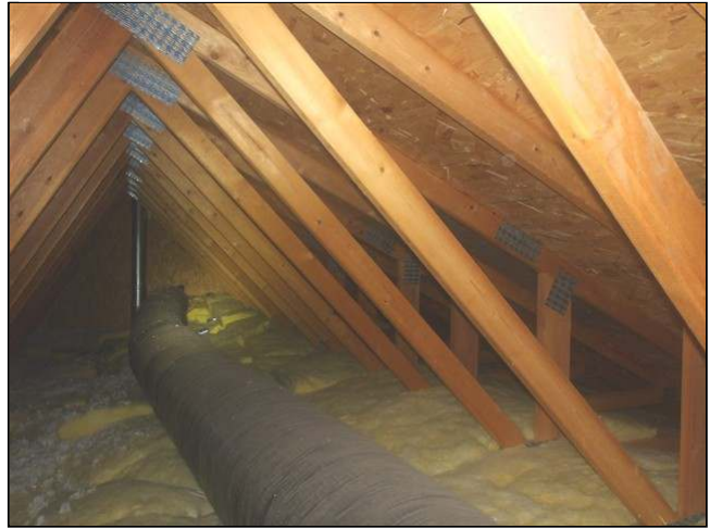
3.8 Item 2(Picture) view of attic
