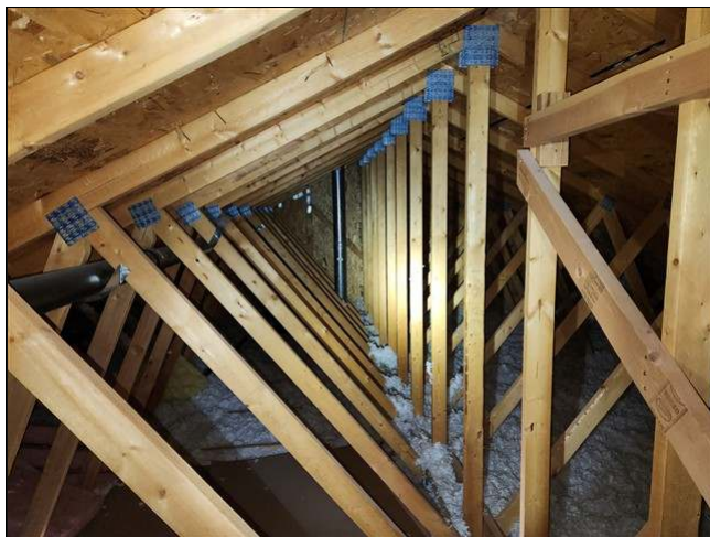
8.11 Item 1(Picture) view of garage roof structure
