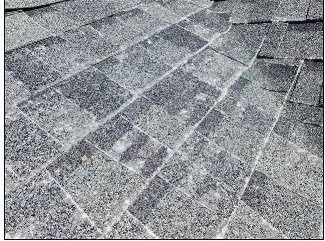
2.1 Item 2(Picture) condition of south shingles
