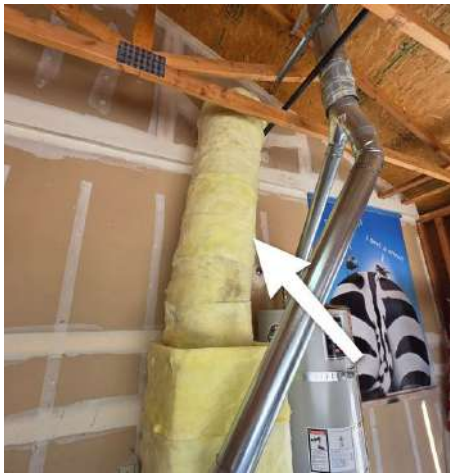
Distribution Systems: Distribution method Insulated
