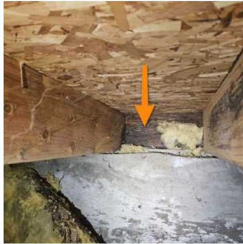
Crawlspace Primary Bathroom
