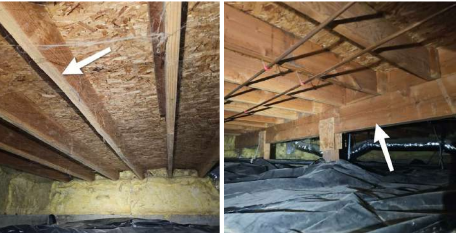
Floor Structure: Material Wood Beams, Wood Floor Joist
