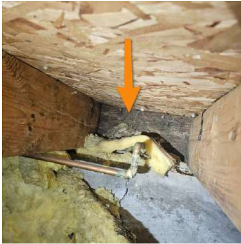
Crawlspace Primary Bathroom
