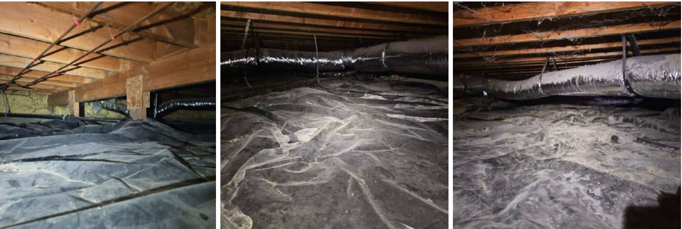
Foundation: Material Concrete
